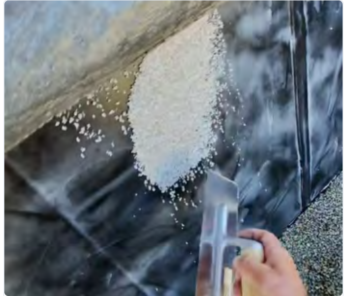
FIG VW.3 Troweling the sand-and-resin charge into the tacky bond coat — top of wall, working downward.
