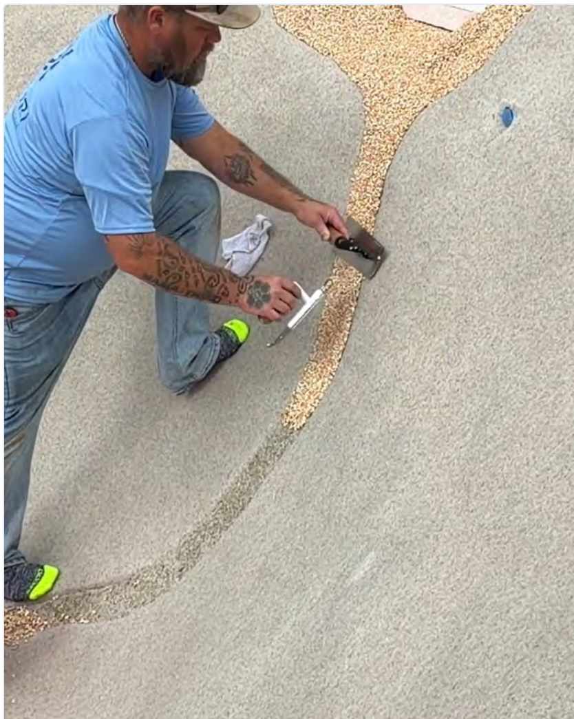
FIG 10.1 Troweling the finishing layer up to a control joint. Maintain clean joint edges and uniform thickness as the layer is consolidated.
