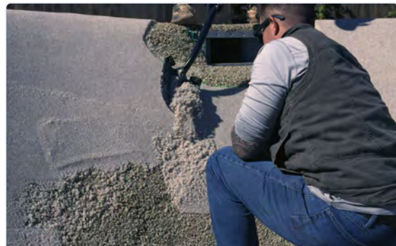
FIG 10.2 Placing finishing-layer aggregate at the work face. Keep batches consistent and place wet-on-wet to avoid cold joints across the lining.
