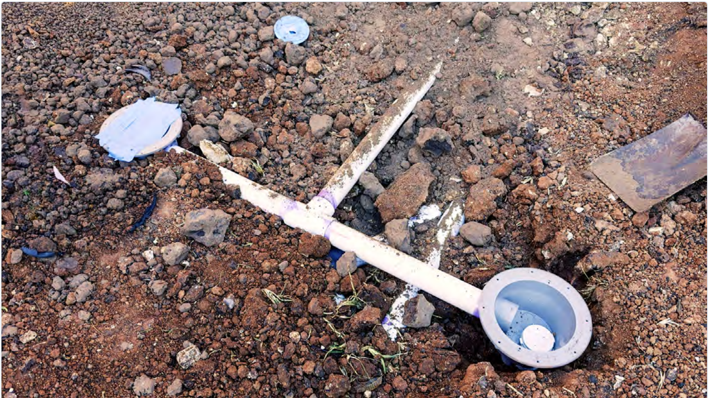
FIG 5.1 Main drain housing with hydrostat valve and delivery pipes set at pool bottom prior to liner installation.
