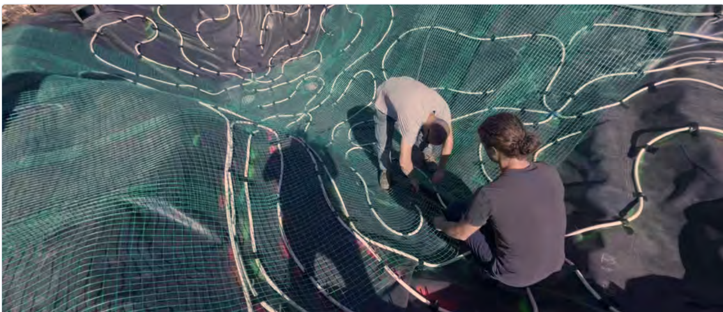
FIG 9.1 Fiberglass mesh laid across the EPDM liner over the spider lines. Sheets overlap by one square (2"); wrinkles are cut and overlapped flat before the base resin lift.
