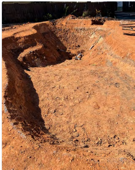
FIG 4.1 Excavation in progress with rounded walls, sloped beach entry, and skimmer pocket cut to reference depths.
