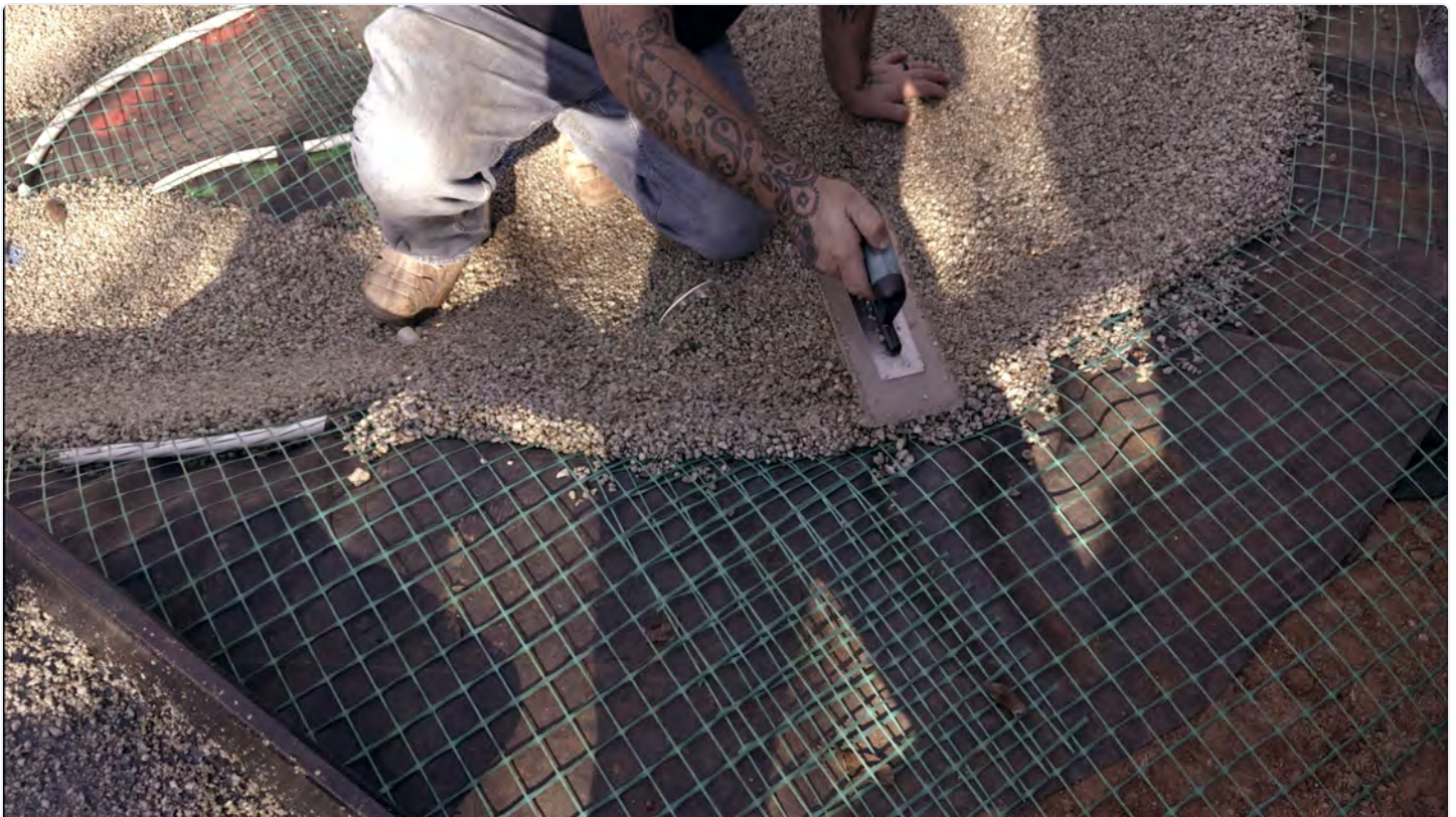
FIG 9.2 Troweling the base resin and crushed-quartz mix over the fiberglass mesh. Aim for a uniform 1½" thickness; if mesh shows through, trim before the next lift.
