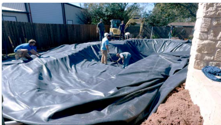
FIG 6.2 Crew positioning the EPDM liner over the protective fabric. Folds are walked out toward the perimeter, then primed and taped before flanging at penetrations.
