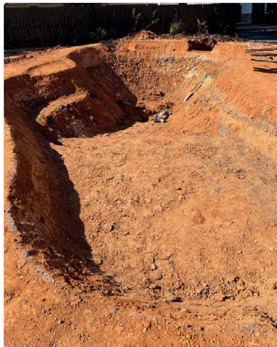
FIG 4.1 Excavation in progress with rounded walls, sloped beach entry, and skimmer pocket cut to reference depths.
