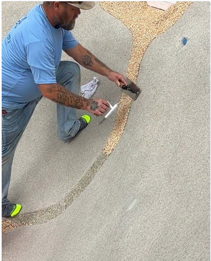
FIG 10.1 Troweling the finishing layer up to a control joint. Maintain clean joint edges and uniform thickness as the layer is consolidated.
