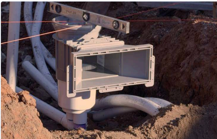
FIG 5.2 Skimmer set 8–13" back from slope edge and leveled with delivery pipes attached (left); collar encased with two 80 lb bags of concrete (right).
