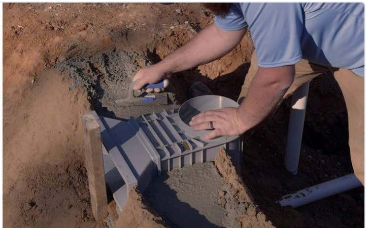
FIG 5.2 Skimmer set 8–13" back from slope edge and leveled with delivery pipes attached (left); collar encased with two 80 lb bags of concrete (right).
