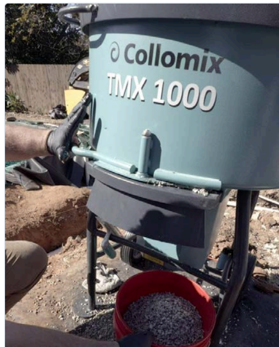
FIG 13.1 Collomix TMX 1000 mixer at the cleaning station. Maintaining a clean drum directly affects color uniformity in the final coat.
