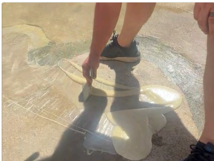
FIG CF.1 Spreading mixed Collaflex across the prepared surface with a trowel. Maintain an even film at the specified coverage rate.
