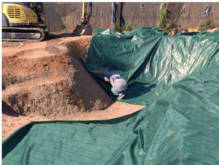
FIG 6.1 Woven protective fabric being laid across the excavated pool surface and dressed into the wall slope before EPDM liner installation.
