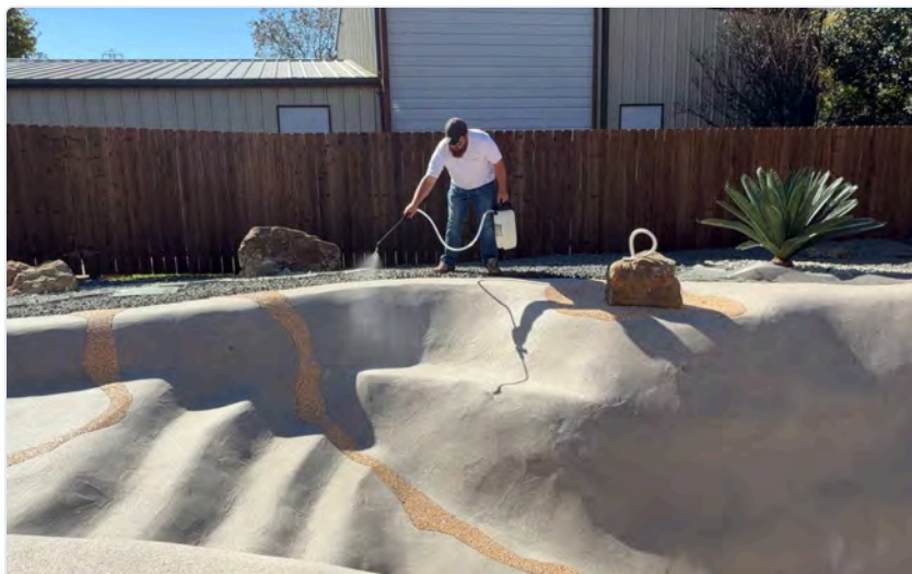
FIG 11.1 Pump-spray application of the final resin sealer over a fully cured, sanded, and dust-free surface. Maintain even passes; avoid pooling on flats.
