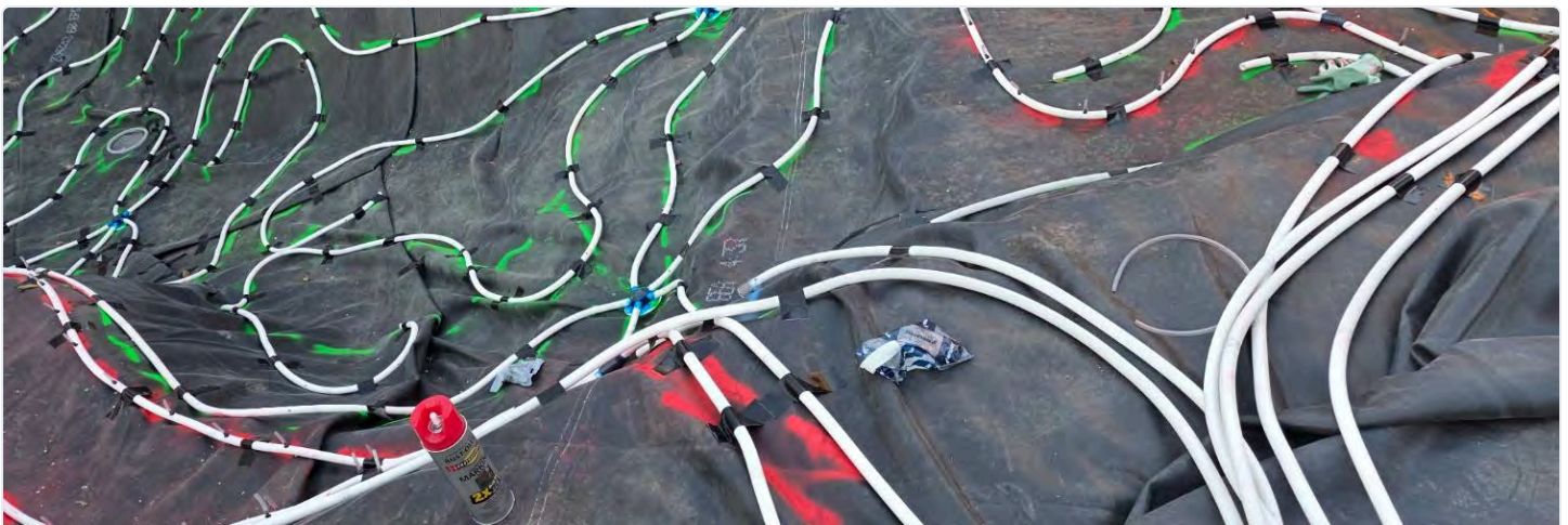
FIG 7.3 Aero-therapy and return-jet lines laid over the EPDM liner. White ½" runs are taped down with chalk-marked routing; lines converge at the distribution box without crossing on open floor.
