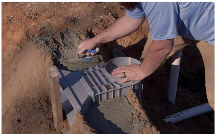
FIG 5.2 Skimmer set 8–13" back from slope edge and leveled with delivery pipes attached (left); collar encased with two 80 lb bags of concrete (right).
