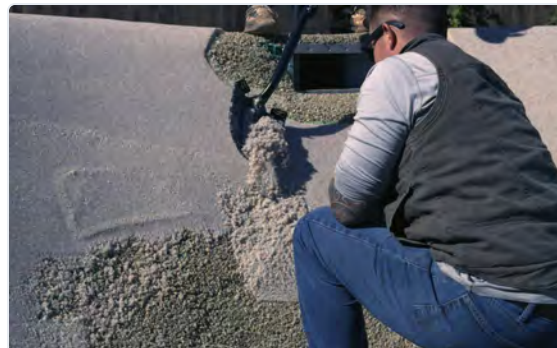
FIG 10.2 Placing finishing-layer aggregate at the work face. Keep batches consistent and place wet-on-wet to avoid cold joints across the lining.
